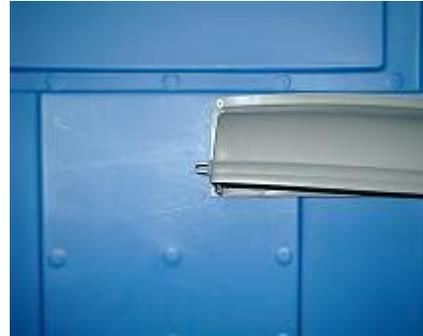
20. Position the door spring guides to the recess in the jamb. Using the provided hole in the spring guide, drill (2) 3/16" holes through first layer of the jamb only. Fasten the top and bottom door spring guide by stretching the cable from the door to the jamb with expanding Rivet #18755 (1) & Washer #11315 (1) on each door spring guide. Check to determine if door catches on roof, by opening door 180° and allowing closing. If roof interferes, remove interfering roof material.
