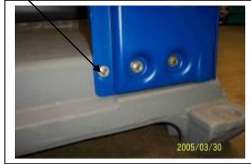
8 Plastic Roto-molded Base. Always tighten the front jambs first with dimples in base. Align jambs to be parallel to the door edge from top to bottom. Then fasten panels to base: start at corners and then center holes. Use screw, #14 x 1-1/2" #13860 (18) and washers, 5/16" #11368 (16). Stop tightening when washer is tight, to avoid stripping out hole.
