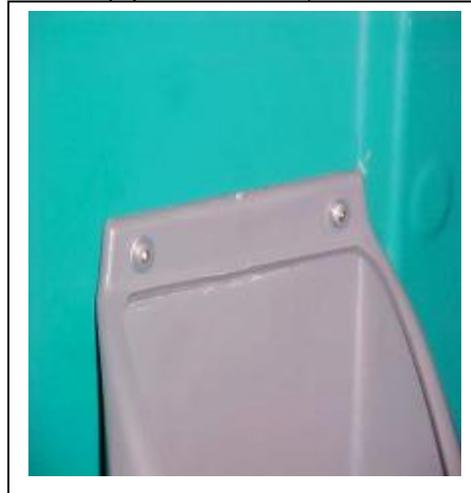
19. Insert the hairpin rod (See fig. A) in the toilet paper holder. Drill (4) 3/16" holes through the toilet paper holder and side wall. The right side of the paper holder should be approximately centered in the front grab area. (See fig. A) The top of the paper holder should be flush with the wall rib just below the signage recess. (See fig. B) Fasten the toilet paper holder with Rivets, #68 AAL #11054 (4) and Washer, 3/16" #11315 (4). Washers are located on the inside of the unit.
